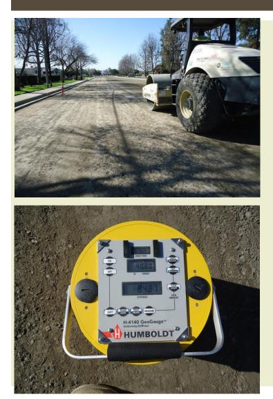
Measure initial stiffness after24 hours of curing
